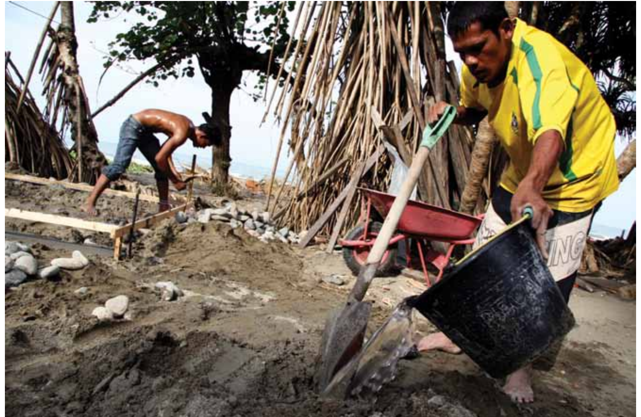
Men at work in Pidie. Photo © UN-Habitat.
