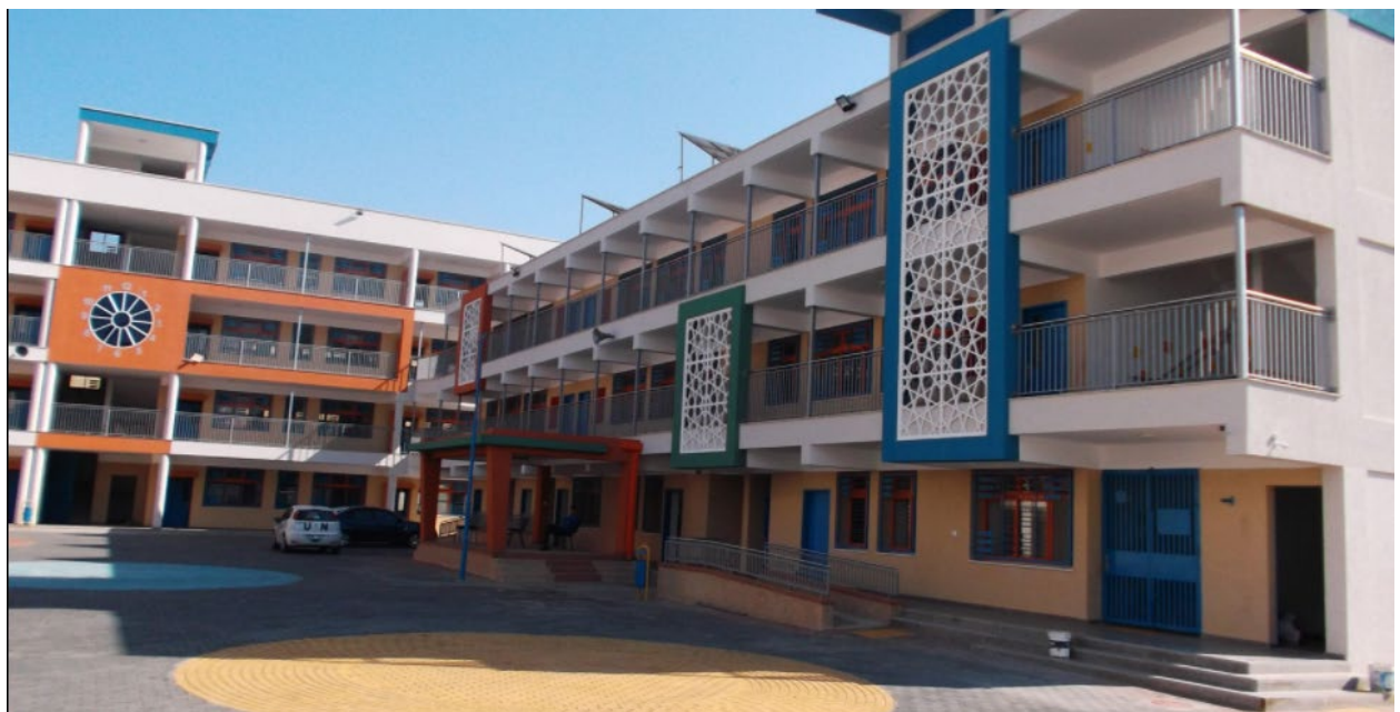
Figure 24: The new UNRWA Gaza elementary coeducational A and B schools. Source: UNRWA (2021).
