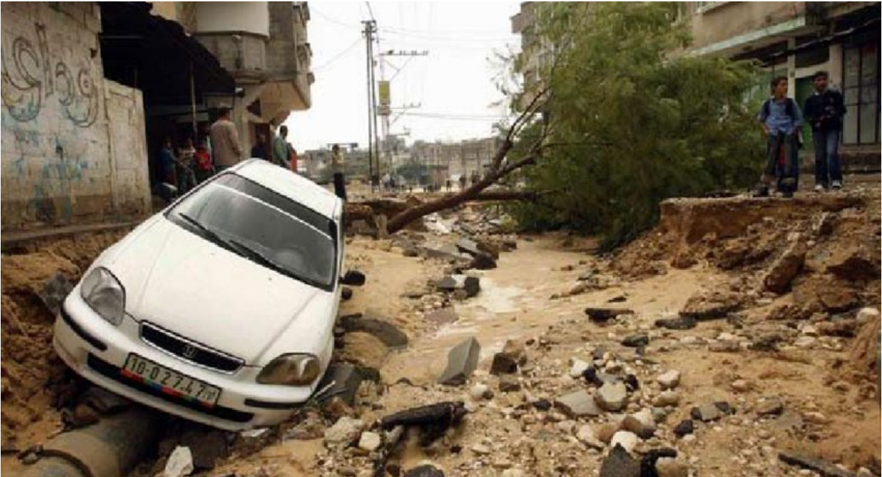
Figure 10: The disruptive and destructive impacts of a flash flood in Gaza 27–29 October 2008. Source: UNDP/PAPP in UNDP (2009).
