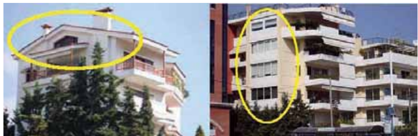
FIGURE 8: Illegal extensions in violation of building regulations; built up “semi-open” areas in new constructions (right) © Dimopoulou & Zentelis, 2008
